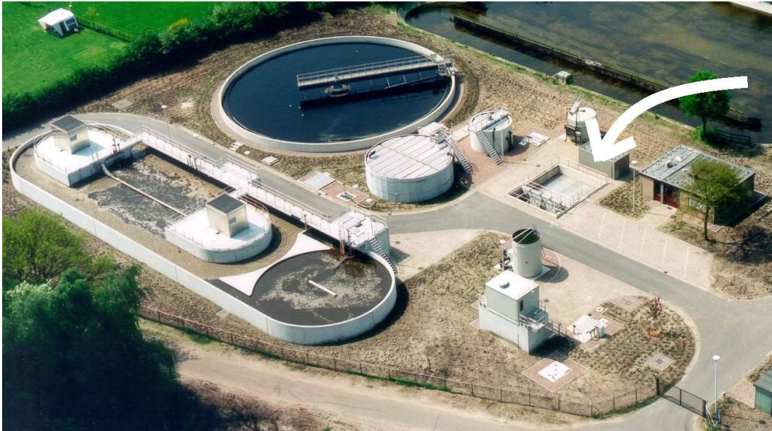
RWZI Ruurlo, filter plant for P removal (1996)
